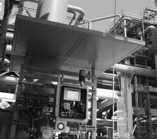
H 2 S IN SOUR GAS — QATAR, 2005
